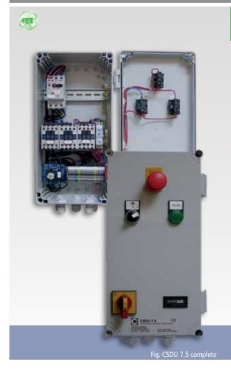
The Condor Pressure Control GmbH CSDU Star/delta connection offers, in due consideration of the relevant standards, the possibility of economically operating motors with a switching capacity greater than 4 kW using public mains networks.
