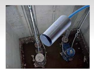
**Level sensor ENS**Monitors e.g. Wastewater/Water level in a pump shaft
